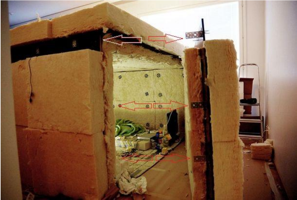
Fastening the door of the capture booth with a nailing angle
